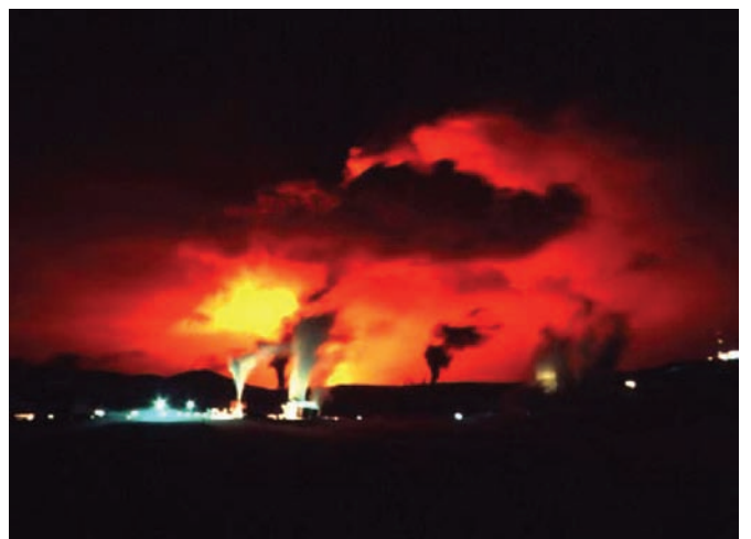
Figure 7 Krafla geothermal power plant during the Krafla fires, 1975–1984. The eruptions slowed down the development of the field for more than 20 years due to volcanic gas contamination of parts of the geothermal field (photo: O. Sigurdsson).
