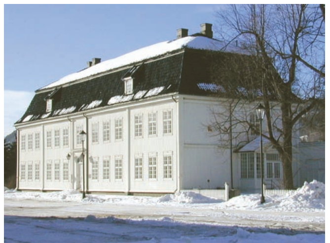
Figure 5 The building of the mining academy – Det Kongelige Norske Berg-Seminarium – at Kongsberg, Norway. The academy, one of the first of its kind, was established in 1757 and associated with the Royal Silver Works. The building is from 1786 and is today part of the Norwegian Museum of Mining. Photo: Norsk Bergverksmuseum, B. I. Berg.
