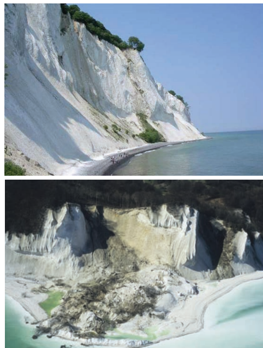
Figure 8 Upper: The chalk cliffs of Møns Klint. Lower: The most recent landslide at Møns Klint, which collapsed in January 2007 (100,000 m 3 chalk created a peninsula 300 m out into the sea) (© SASP).
